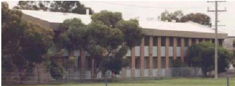
Comalco Research & Technology Buildings, Victoria Insultec applied Sections 1 and 2, January & July 1994.
